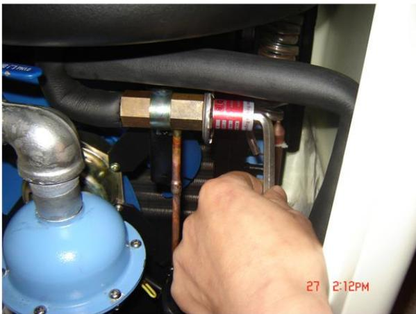
*Turn the valve clockwise slowly with the 8mm hex key wrench until the E.V.TEMP shows the pressure 38psi~42psi.*
